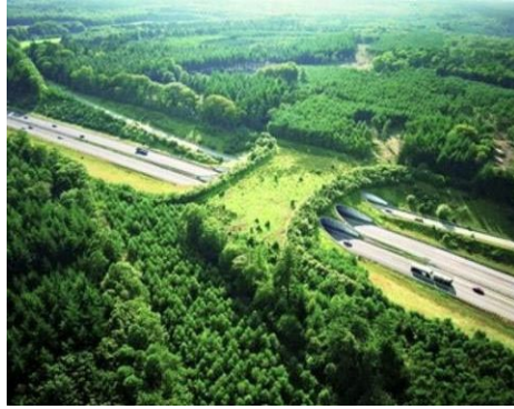
Biodiversity bridge Netherlands cc)
